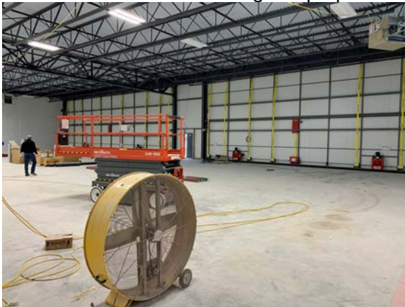
Interior photo of the hangar space.
