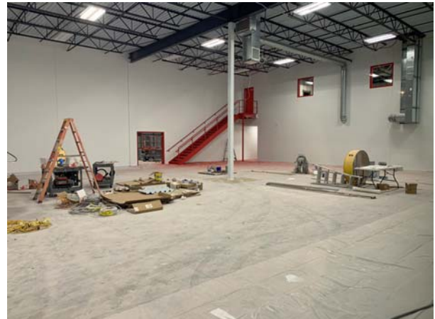
Interior photo of workshop – nearing completion
