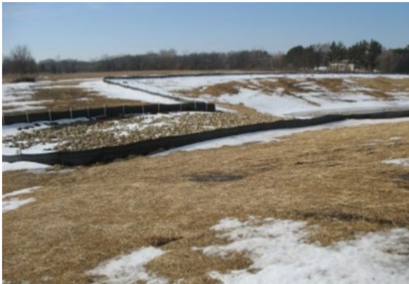
Silt fence used as perimeter control
