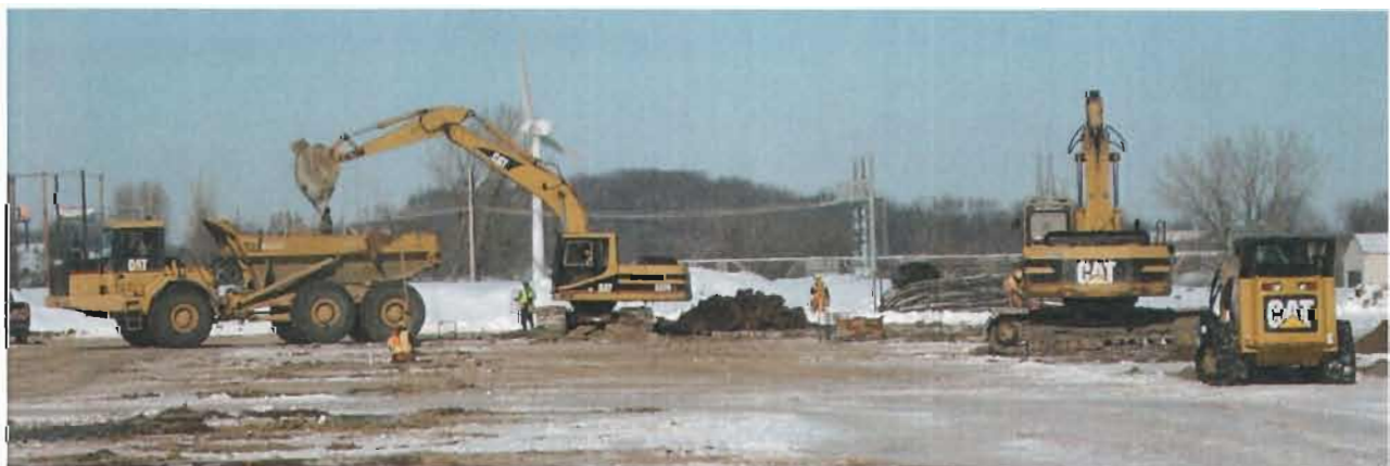
Construction site for SAGE Electrochromics, Inc.
