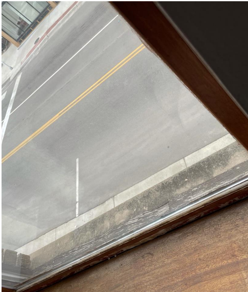
Existing window to be replaced – on south façade of building.
