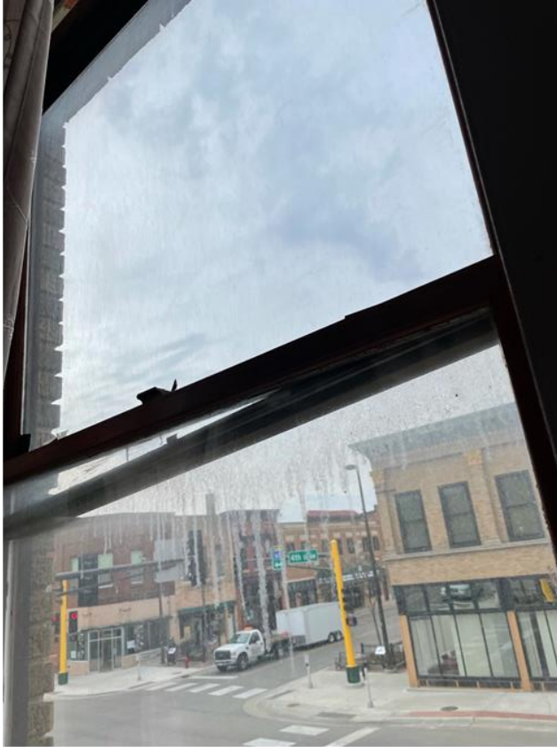
View of inside of window – on south façade of building.
