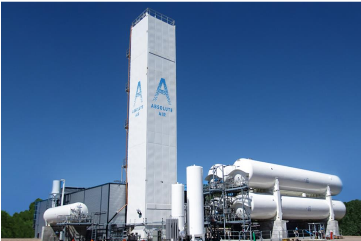
Example of a Typical Air Separation Plant
