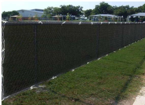
Example of 6' chain link with mesh screen (not allowed for residential uses)
